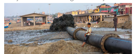
► Dredging at Thankasseri, 2014, Photo: Jishnu S. Chandran, KCHR
